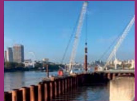
Local residents and businesses will be pleased to hear that with the last of the long piles successfully inserted on October 22nd, noisy percussive piling has now been completed at the Blackfriars Bridge Foreshore site. Going forward Tideway will be inserting sheet piles in the eastern cofferdam using the quieter vibro method.
