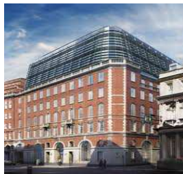
67 Lombard St completed 2013
