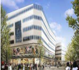
One New Change completed 2011
