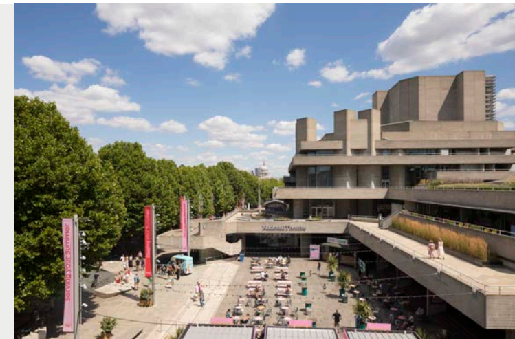
f17 | Waterloo Bridge downstream - overlooking terraces of RNT
