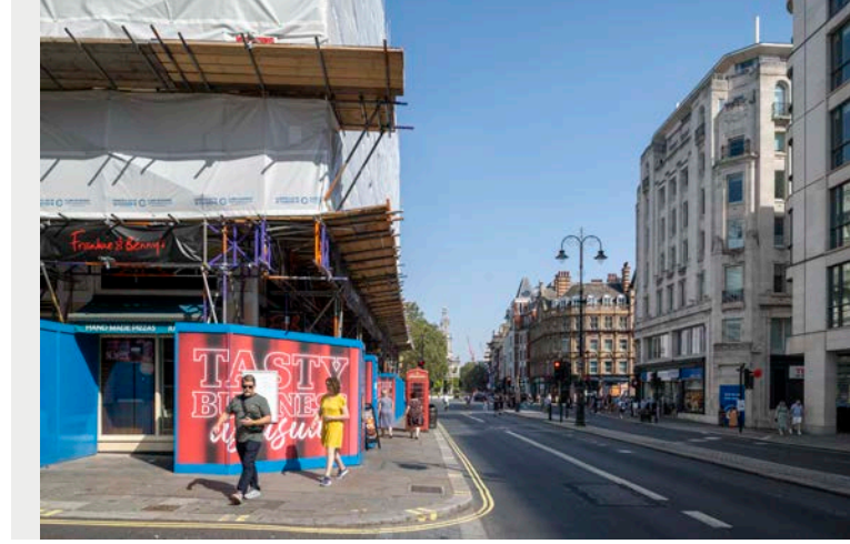
f26 | The Strand west, at Burleigh Street - north pavement
