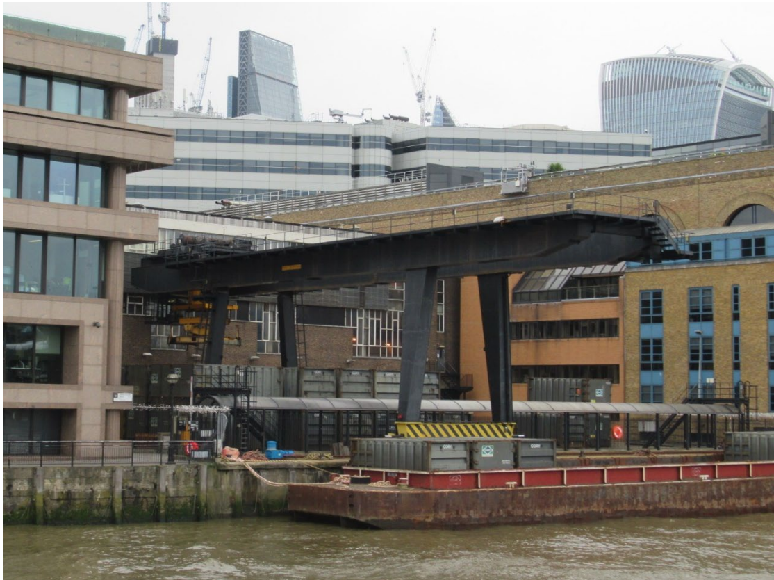
Walbrook Wharf Waste Transfer Station
