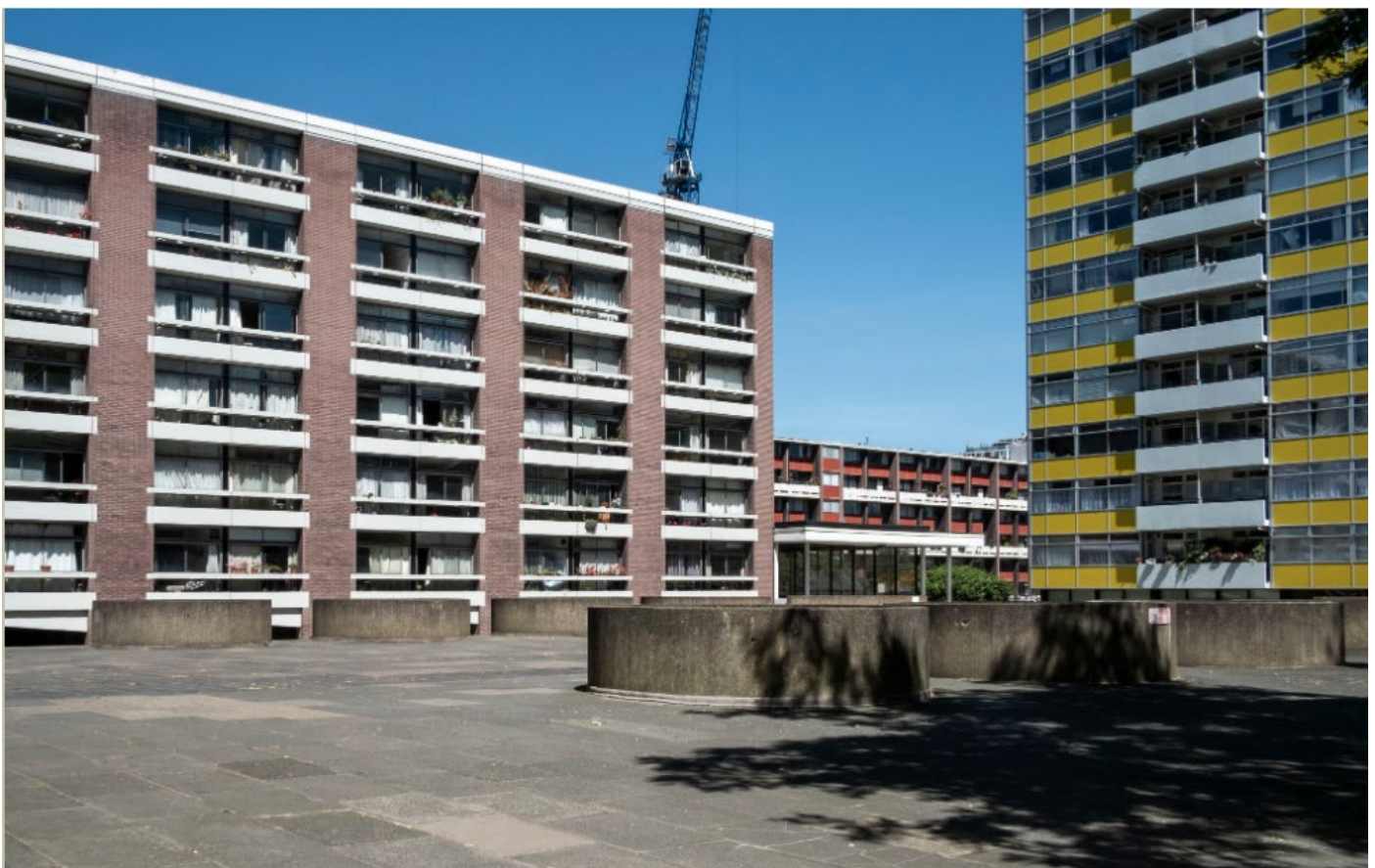
Looking towards Cullum Welch House (L) and Great Arthur House (R), with Basterfield House glimpsed in the distance
