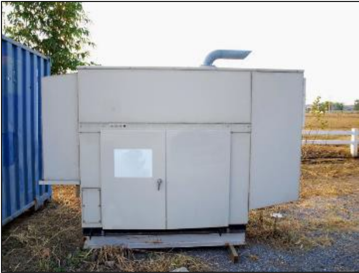
Figure 4-2: Example generator plant with horizontal discharge
