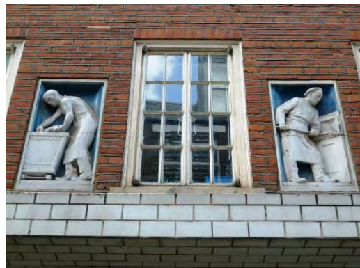
12-13 Widegate Street (former bakery)
