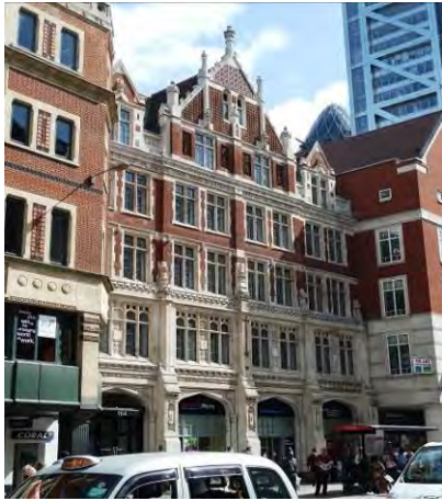
Former Fire Brigade Station
