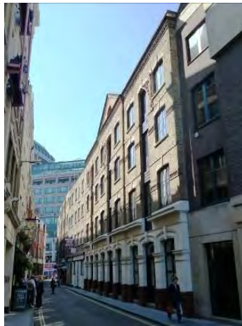
Artillery Lane, north side
