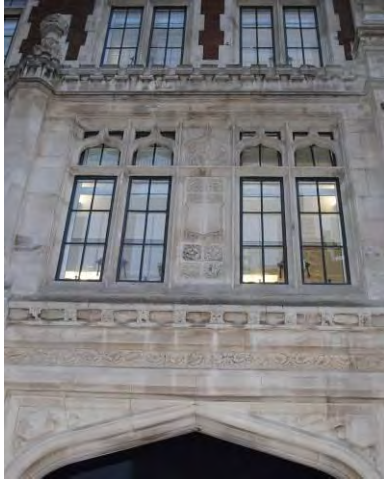
Former Fire Brigade Station
