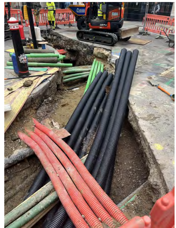
The new ductwork being installed amongst existing infrastructure beneath the highway
