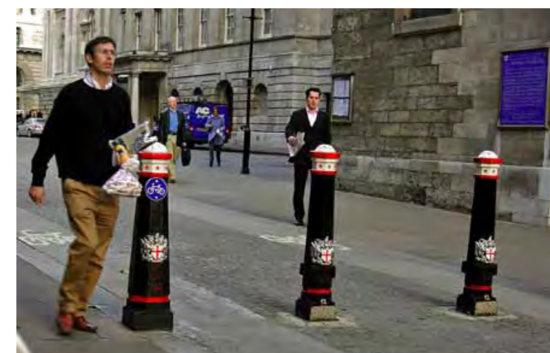
Bollard line with C3 demountable bollards
