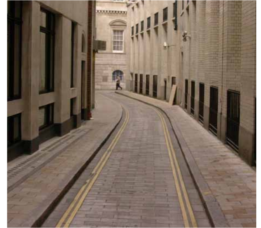
Retained raised kerb to carriageway
