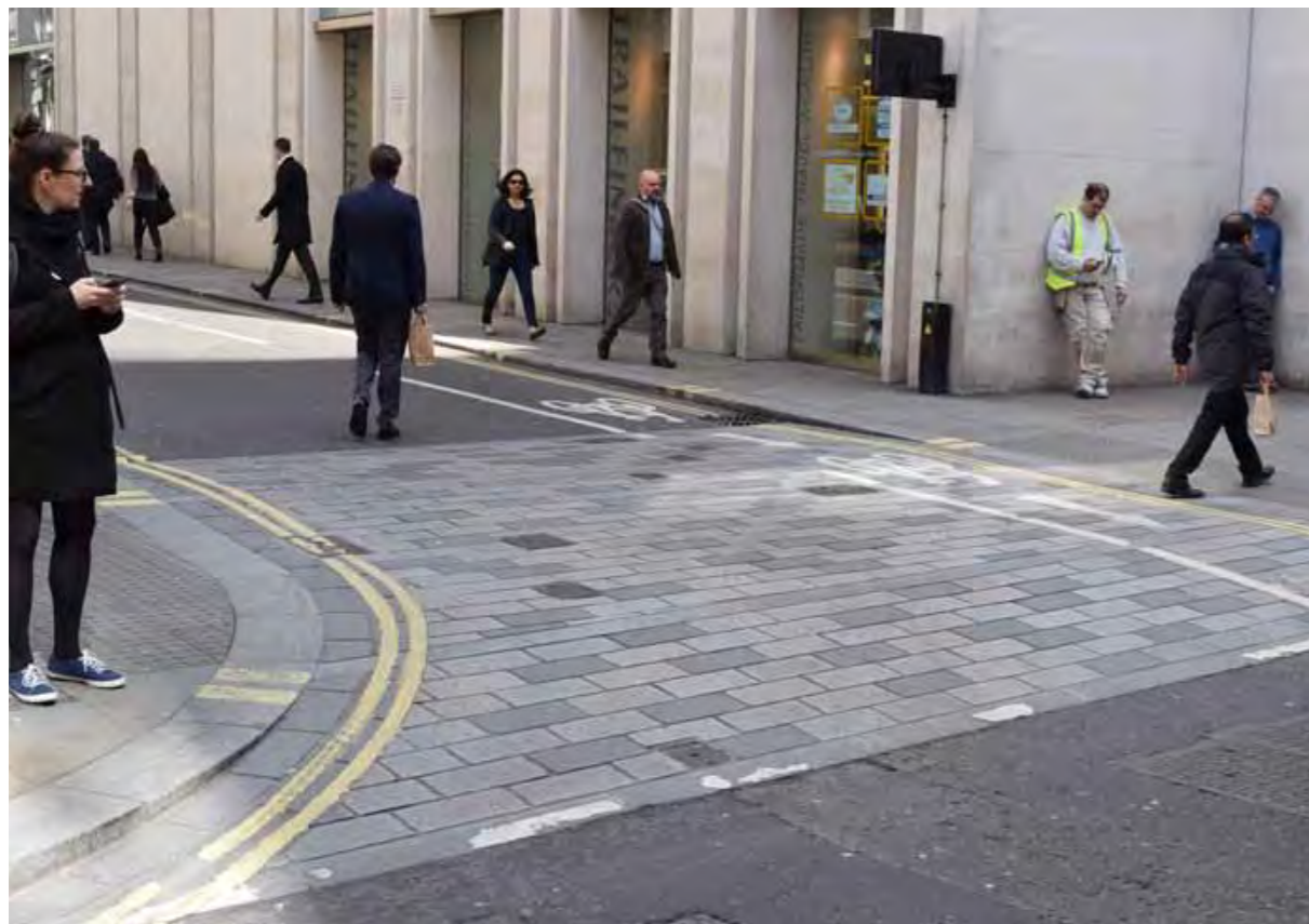
Granite setted courtesy crossing
