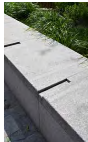
Groove cut into stone
