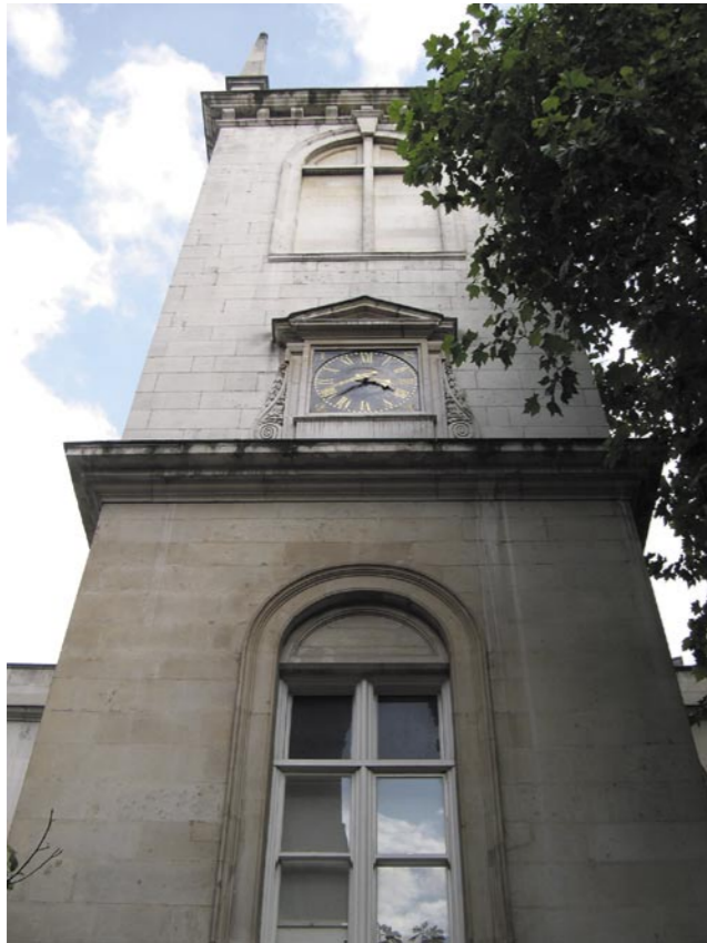
Tower of former Church St Olave
