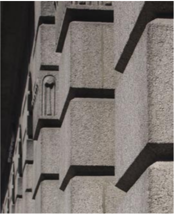
Columns, Atlas building King Street
