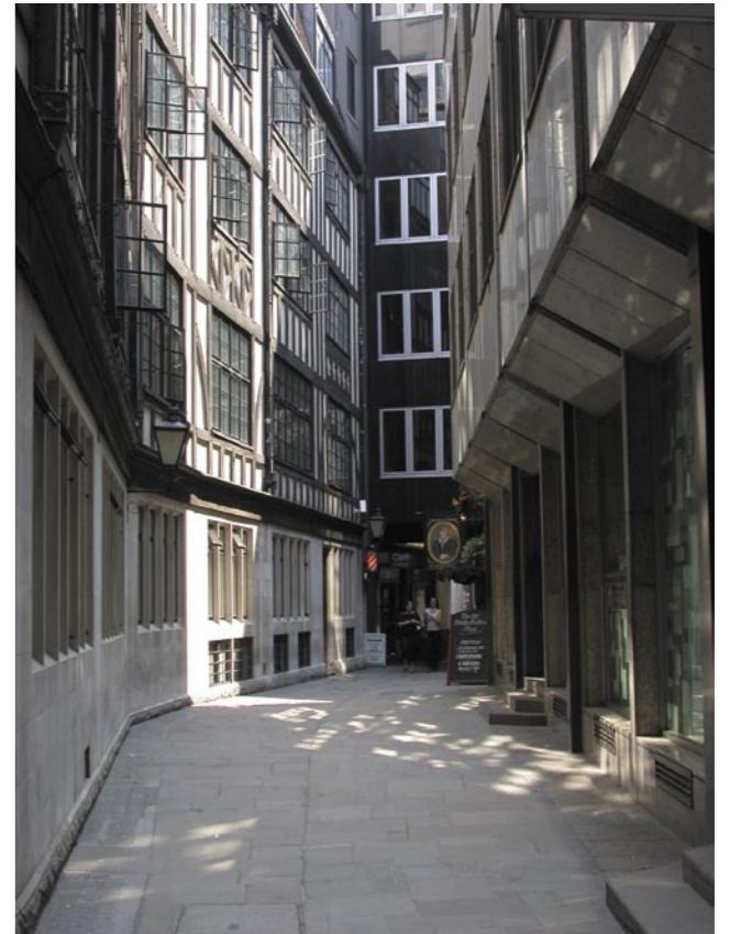
Masons Avenue, looking east
