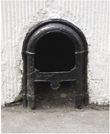
Foot scraper, Old Jewry
