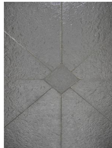
New Caithness stone paving at Guildhall entrance
