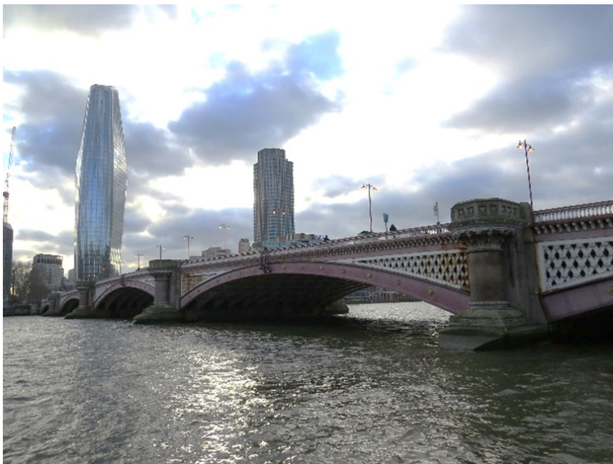
Picture 1: Blackfriars Bridge
