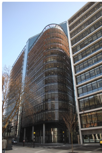
Photo 29: 1 New Street Square
