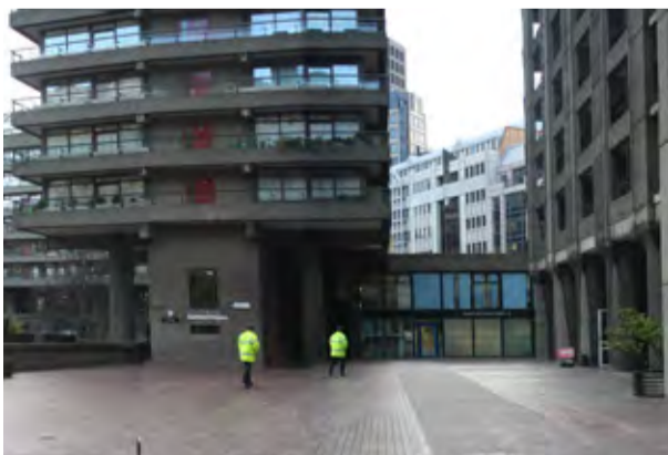
View of Lauderdale Place, looking south. The blank frontage of the Barbican estate office can be seen straight ahead, with the shop located on the ground floor of Lauderdale Tower just seen on the right.
