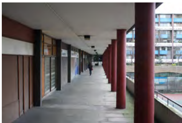
View showing the eastern façade of retail units in Crescent House, facing into the Golden Lane estate (looking north). These shops were designed with an eastern and western entrance, but the majority of occupiers have only retained western access from Goswell Road, with interior layouts oriented towards this street. Consequently, views into most units from the east are severely obstructed, or reveal storage and back-office areas. As a result the adjacent space is of poor quality with little activation
