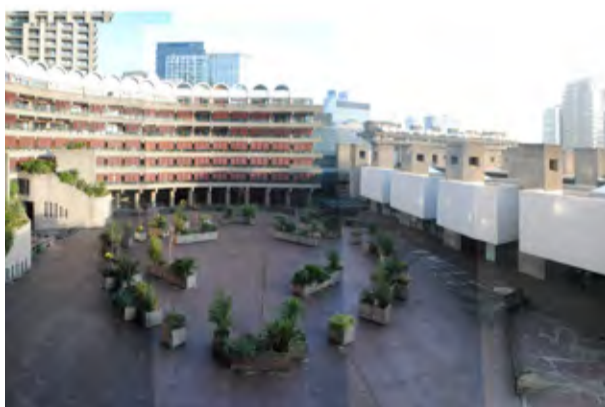
Frobisher Court and the Barbican Art Gallery's unused entrances (above right), seen from above, looking east. The space is currently poorly connected to surrounding buildings and other parts of the podium. Although adjacent, the Barbican Centre and its art gallery have little relationship with Frobisher Court
