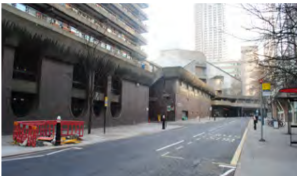
View along Silk Street looking west towards the GSMD and Barbican Centre. The street's southern edge is dominated by car parks and it currently hosts little street-level activity. During the evening (a time when many visitors attend concerts and cultural events in the area) lighting within the car parks increases their prominence, to the detriment of the public realm. Cultural uses along Silk Street have little presence in the public realm and although the GSMD's main entrance is located here, it is difficult to distinguish, particularly from a distance
