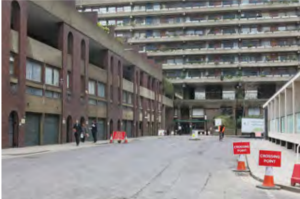
View looking north along Wood Street. The route into the Barbican estate via St Giles' Terrace and access points onto the highwalk network are difficult to discern from a distance
