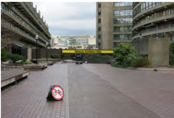
The 'Yellow Shed', seen from Ben Jonson Place on the upper podium (looking east). Although prominently signed, this entrance to the Barbican Exhibition Halls is not in use, and obstructs views and permeability across the upper podium
