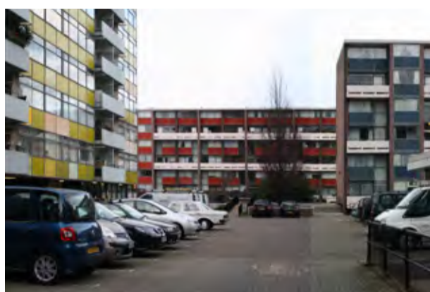
View of the eastern forecourt of Great Arthur House, looking north. The space is currently dominated by parked cars
