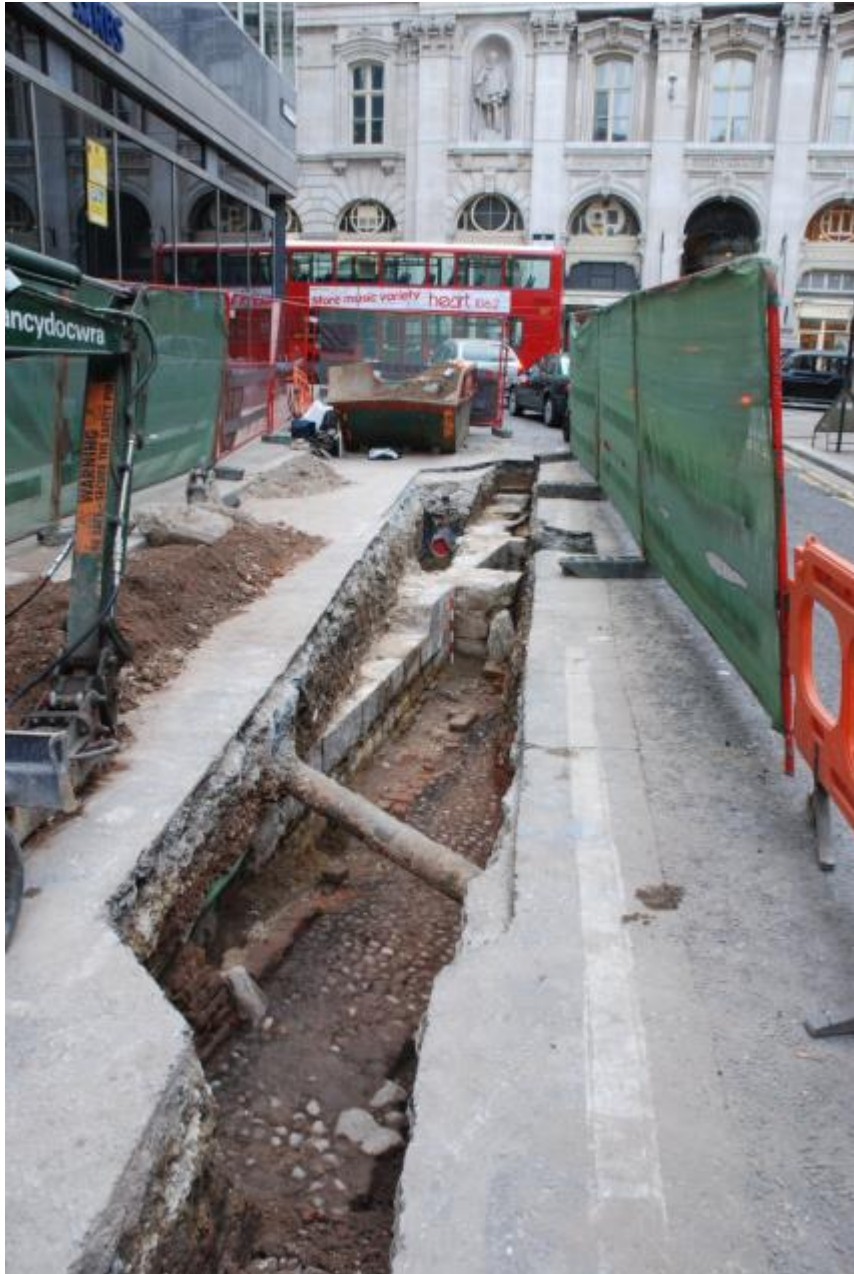
Bartholomew Lane, Thames water main replacement: © Compass Archaeology
