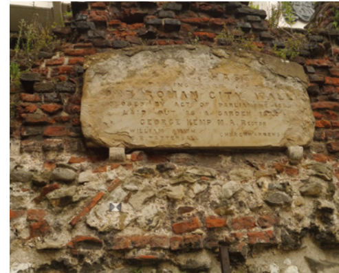
The Roman City wall and its top layer of bricks from 1477 at St Alphege Garden
